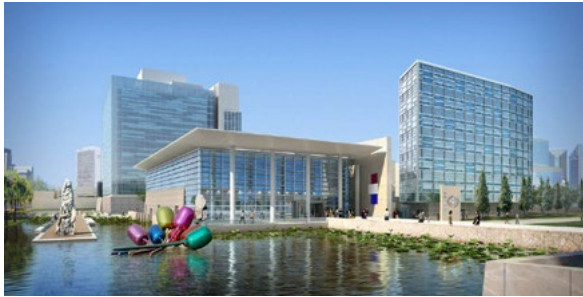
Skidmore, Owings and Merrill, LLP
